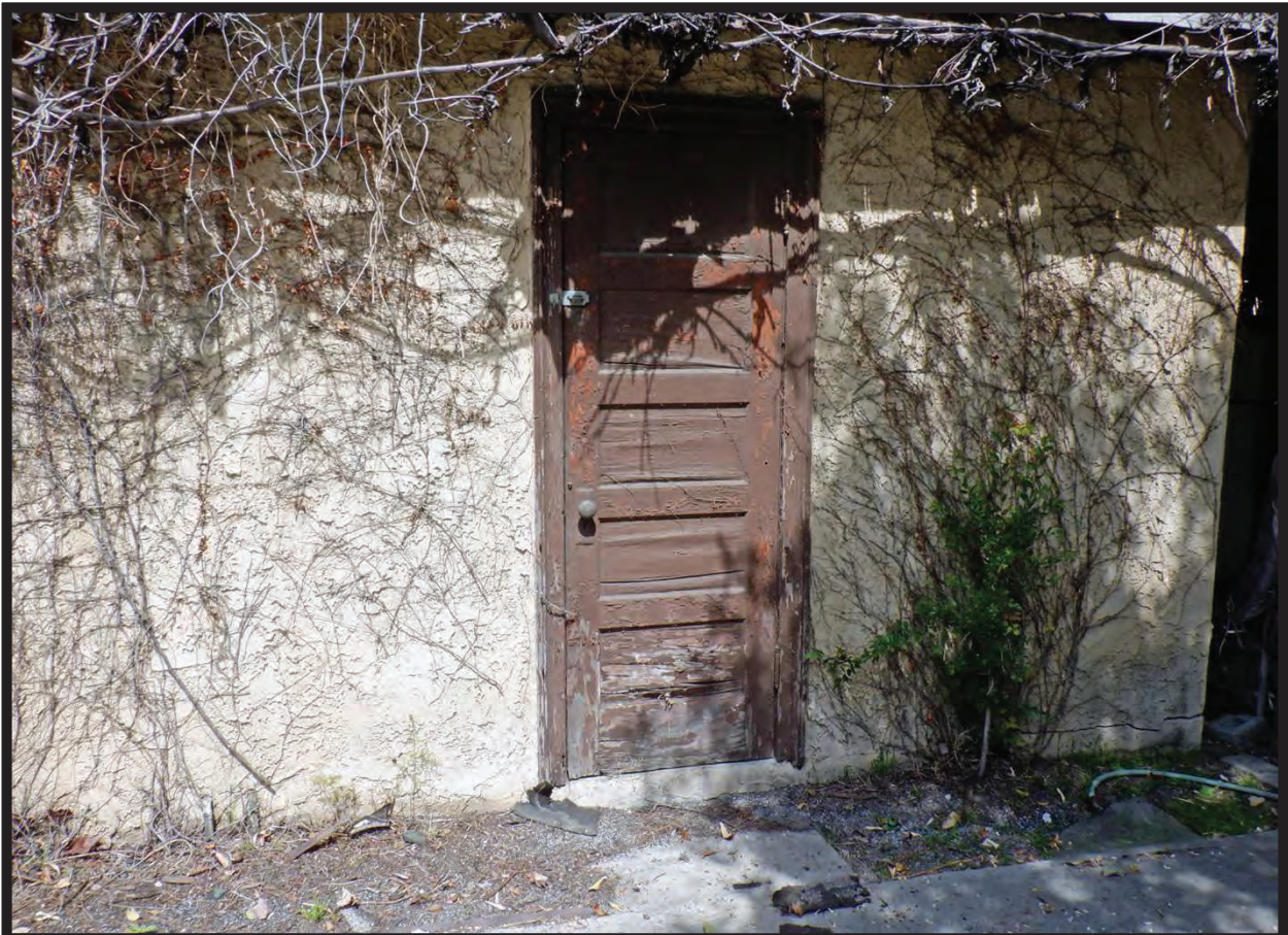
South Elevation of 1926-1927 Garage, 1022 La Cadena Avenue, Arcadia, CA (N)
