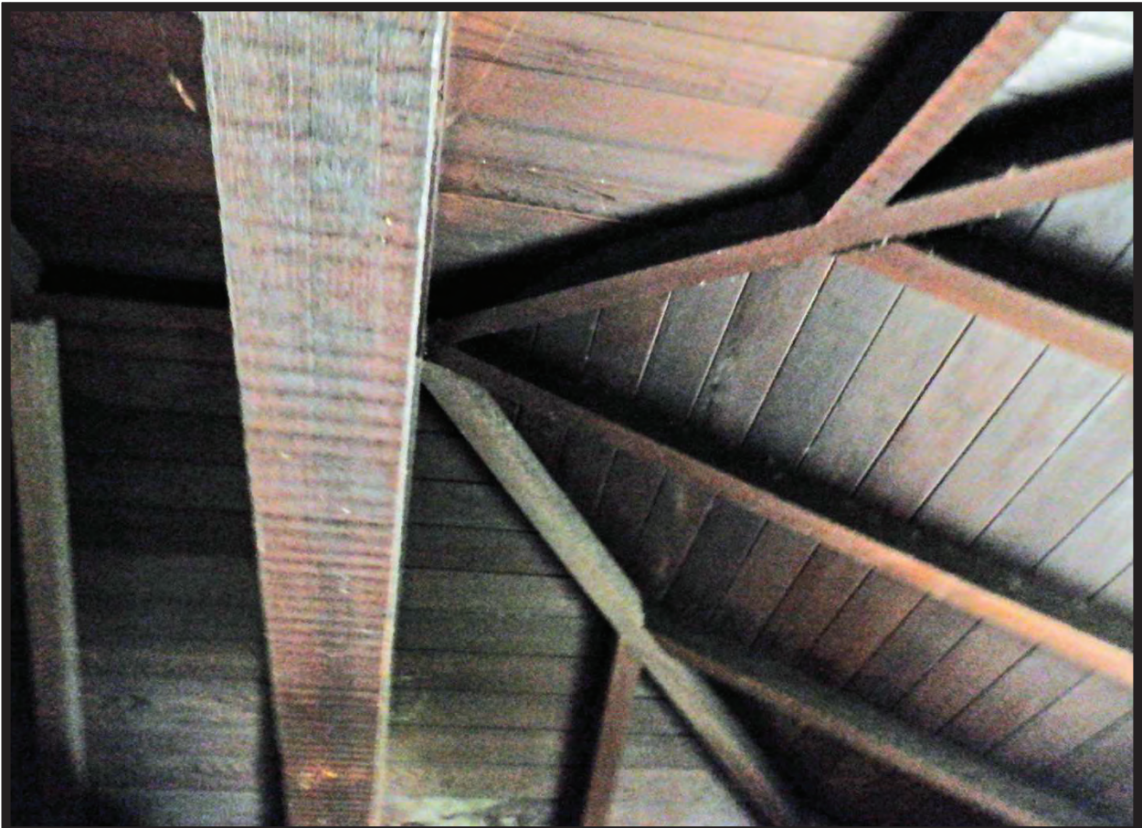
Interior of 1944 Residence at 1022 La Cadena Avenue, Arcadia, CA (S)
