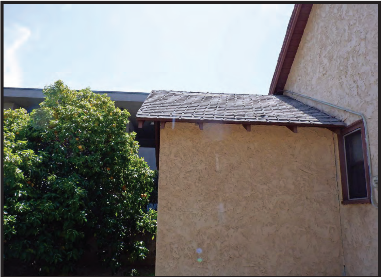
Addition on East Elevation of Residence at 1022 La Cadena Avenue, Arcadia, CA (S)
