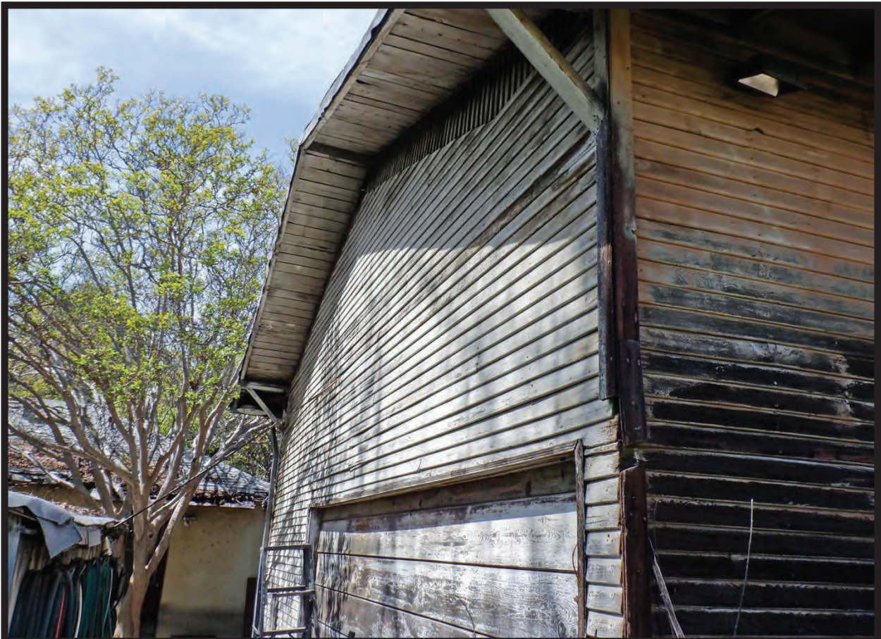
South Elevation of Large Barn/Workshop with Bay Door, 1022 La Cadena Avenue, Arcadia, CA (WNW)
