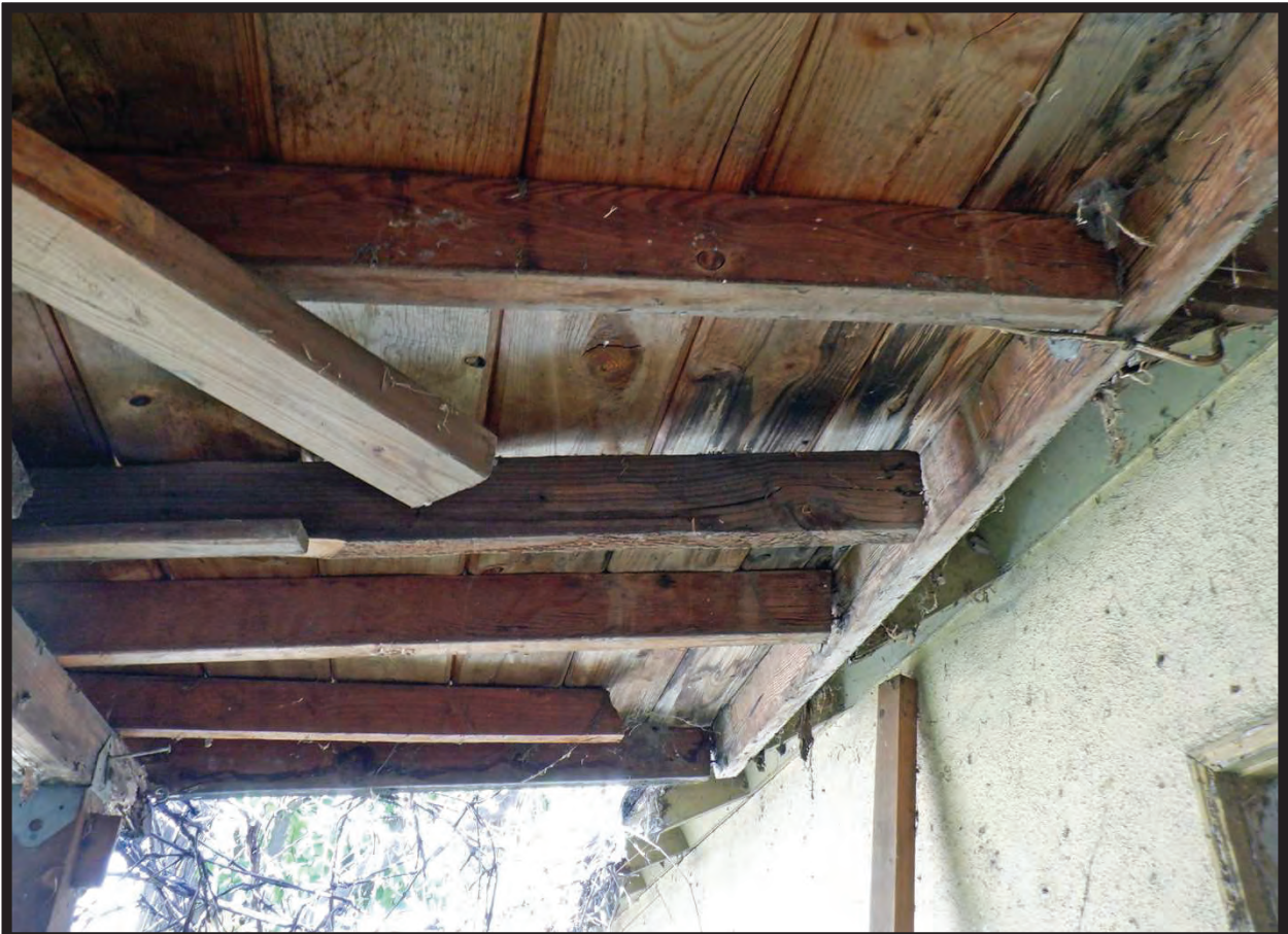
Added Roofing North of 1944 Residence at 1022 La Cadena Avenue, Arcadia, CA (ESE)
