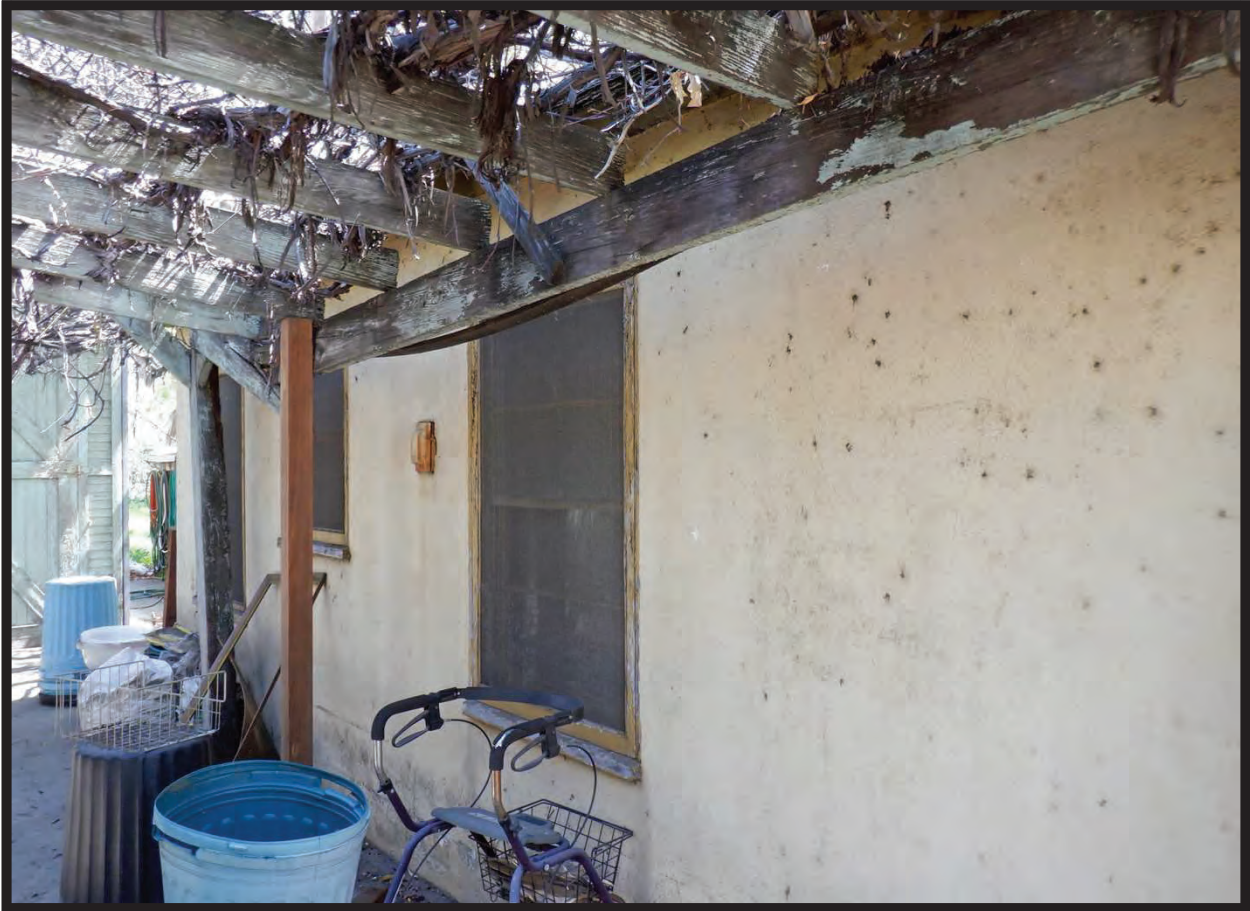
North Elevation of 1944 Residence at 1022 La Cadena Avenue, Arcadia, CA (ESE)
