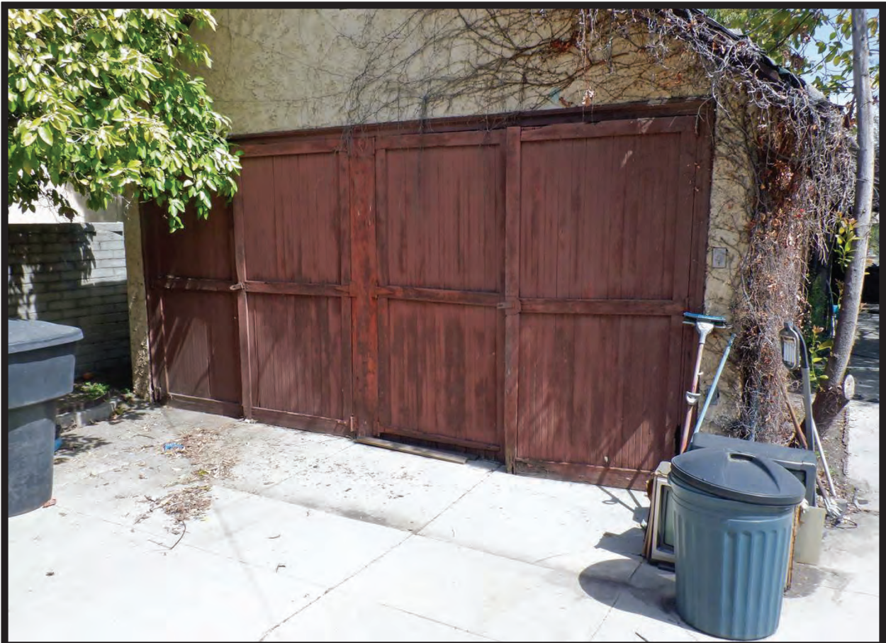
West Elevation of 1926-1927 Garage, 1022 La Cadena Avenue, Arcadia, CA (ENE)
