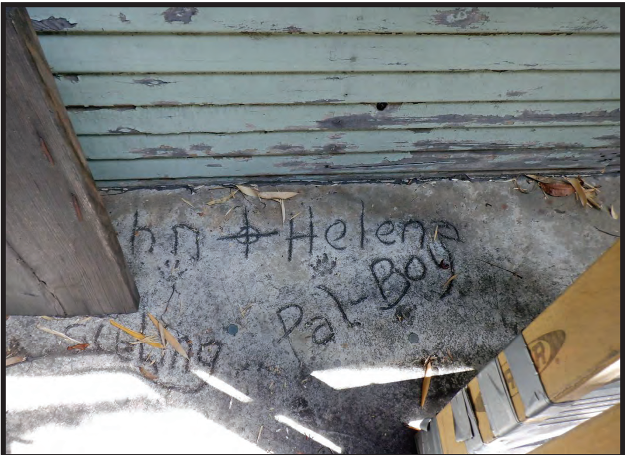
Markings in Concrete to West of Office, 1022 La Cadena Avenue, Arcadia, CA (Detail)
