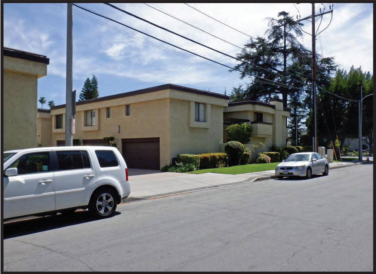
Residences at 479-489 W. Duarte Road, Arcadia, CA (MFR, 1974; SE)
