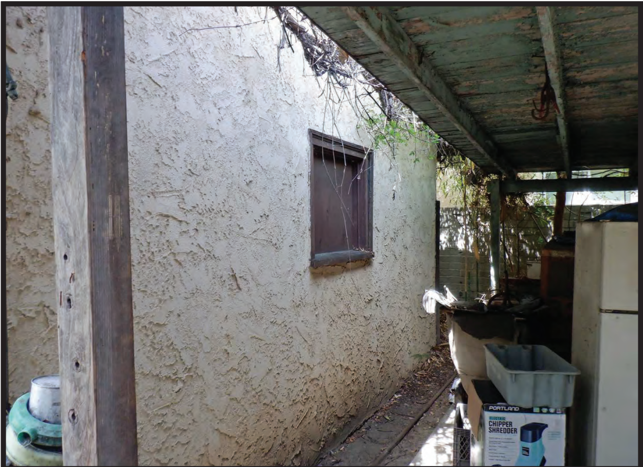
East Elevation of 1926-1927 Garage, 1022 La Cadena Avenue, Arcadia, CA (NNW)
