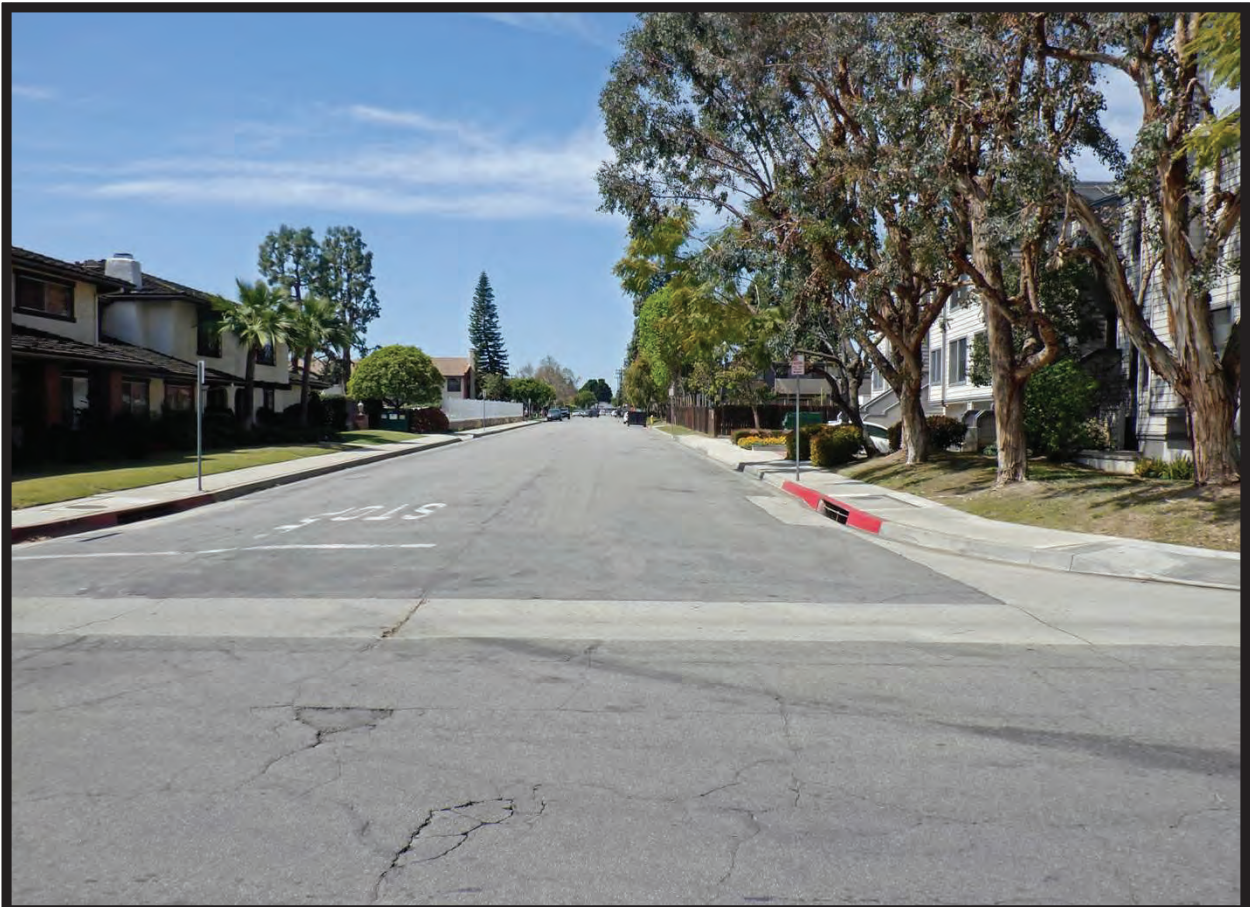
Overview of Arcadia Avenue from La Cadena Avenue, Arcadia, CA (W)
