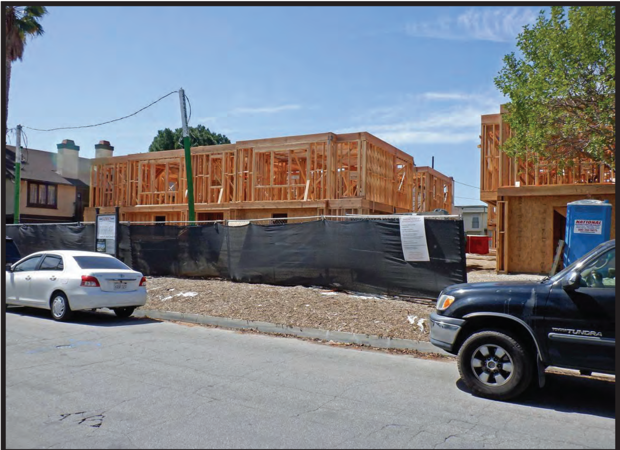
Property Under Construction at 1111-1117 La Cadena Avenue, Arcadia, CA (MFR, WSW)
