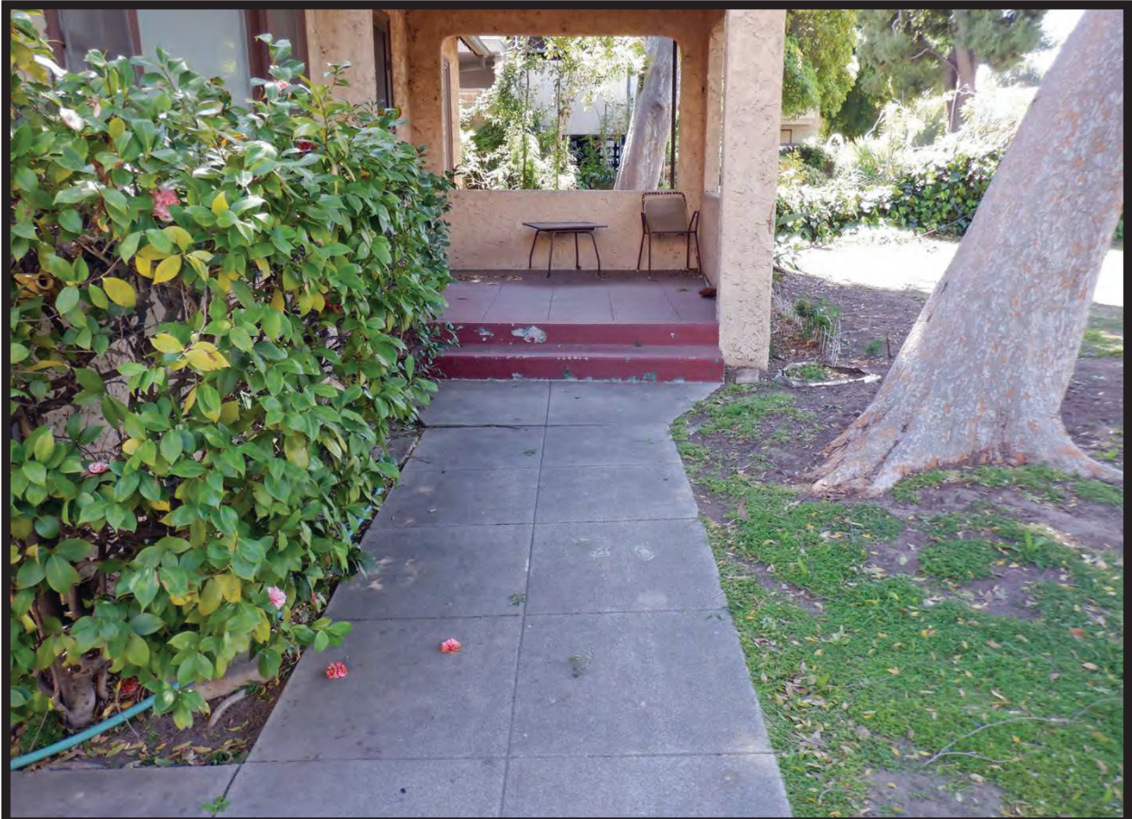
Porch on West Elevation of Residence at 1022 La Cadena Avenue, Arcadia, CA (S)
