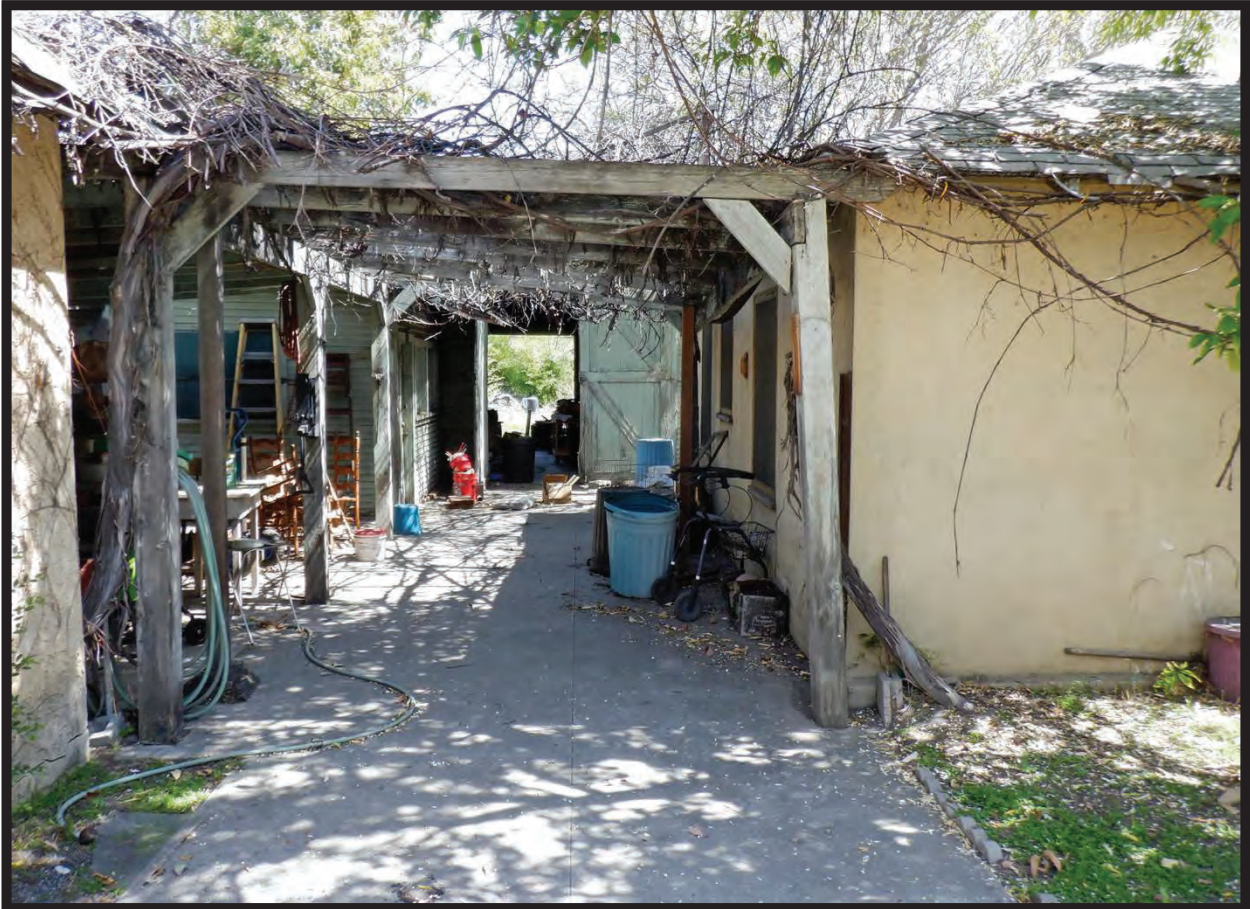
Paved Alignment between Garage and 1944 Residence at 1022 La Cadena Avenue, Arcadia, CA (E)
