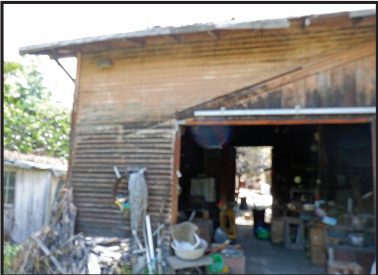
East Elevation of Large Barn/Workshop, 1022 La Cadena Avenue, Arcadia, CA (WSW)
