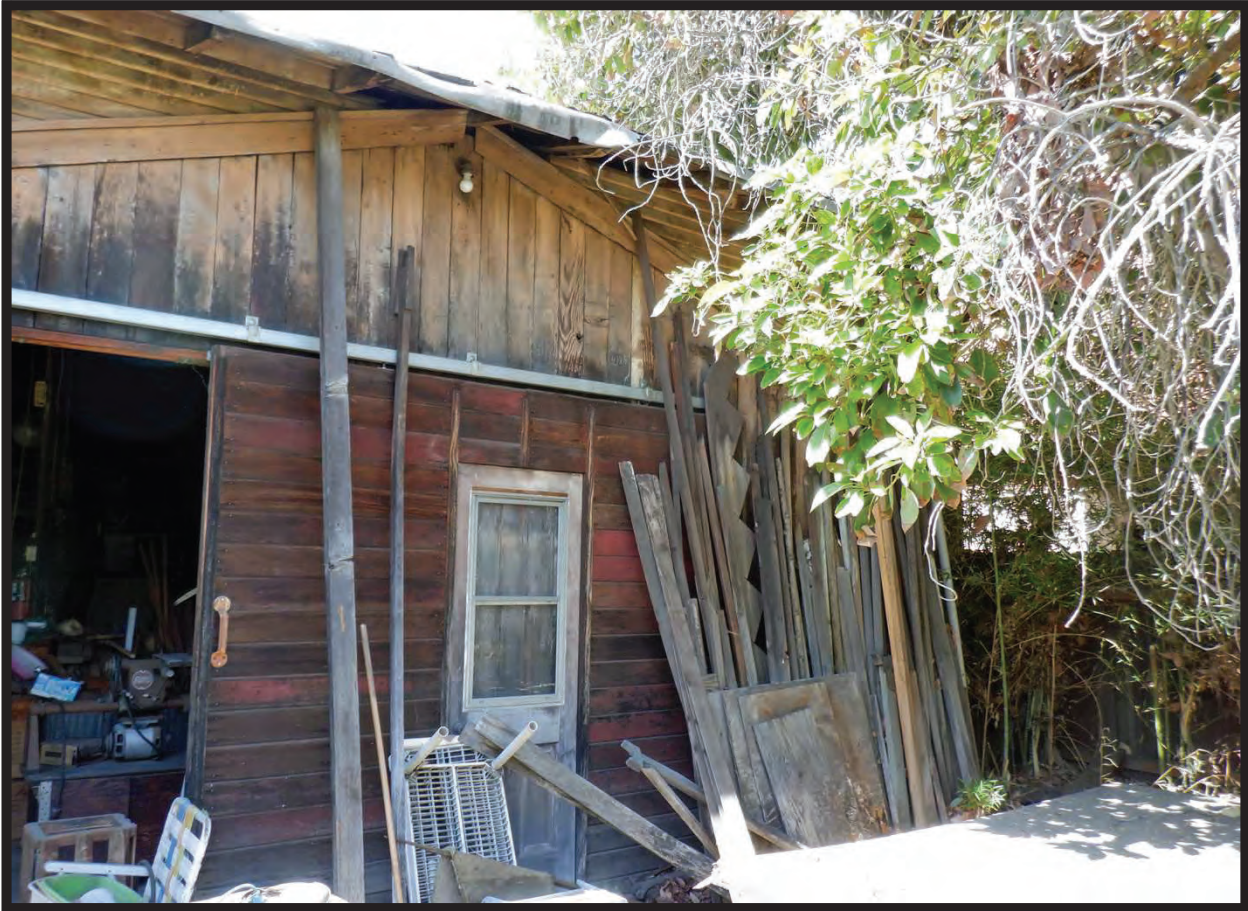
East Elevation of Large Barn/Workshop, 1022 La Cadena Avenue, Arcadia, CA (NW)
