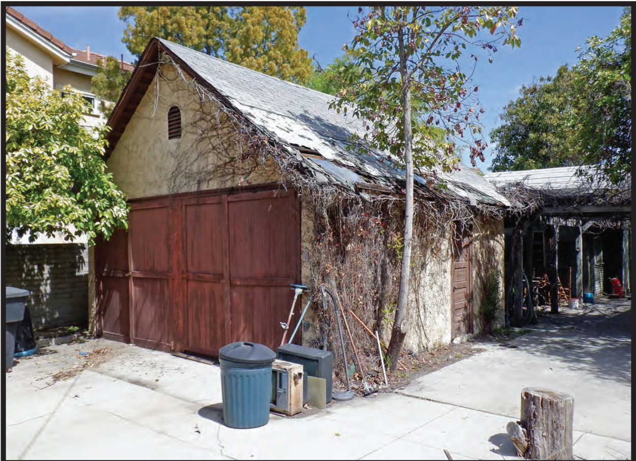
Overview of 1926-1927 Garage, 1022 La Cadena Avenue, Arcadia, CA (NE)
