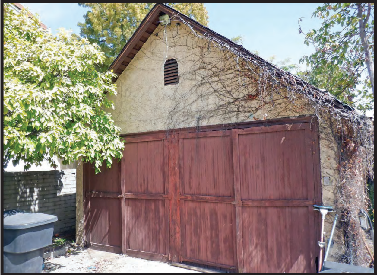
West Elevation of 1926-1927 Garage, 1022 La Cadena Avenue, Arcadia, CA (NE)
