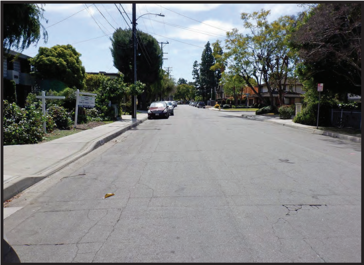
Overview of La Caden Avenue, towards Duarte Road, Arcadia, CA (S)
