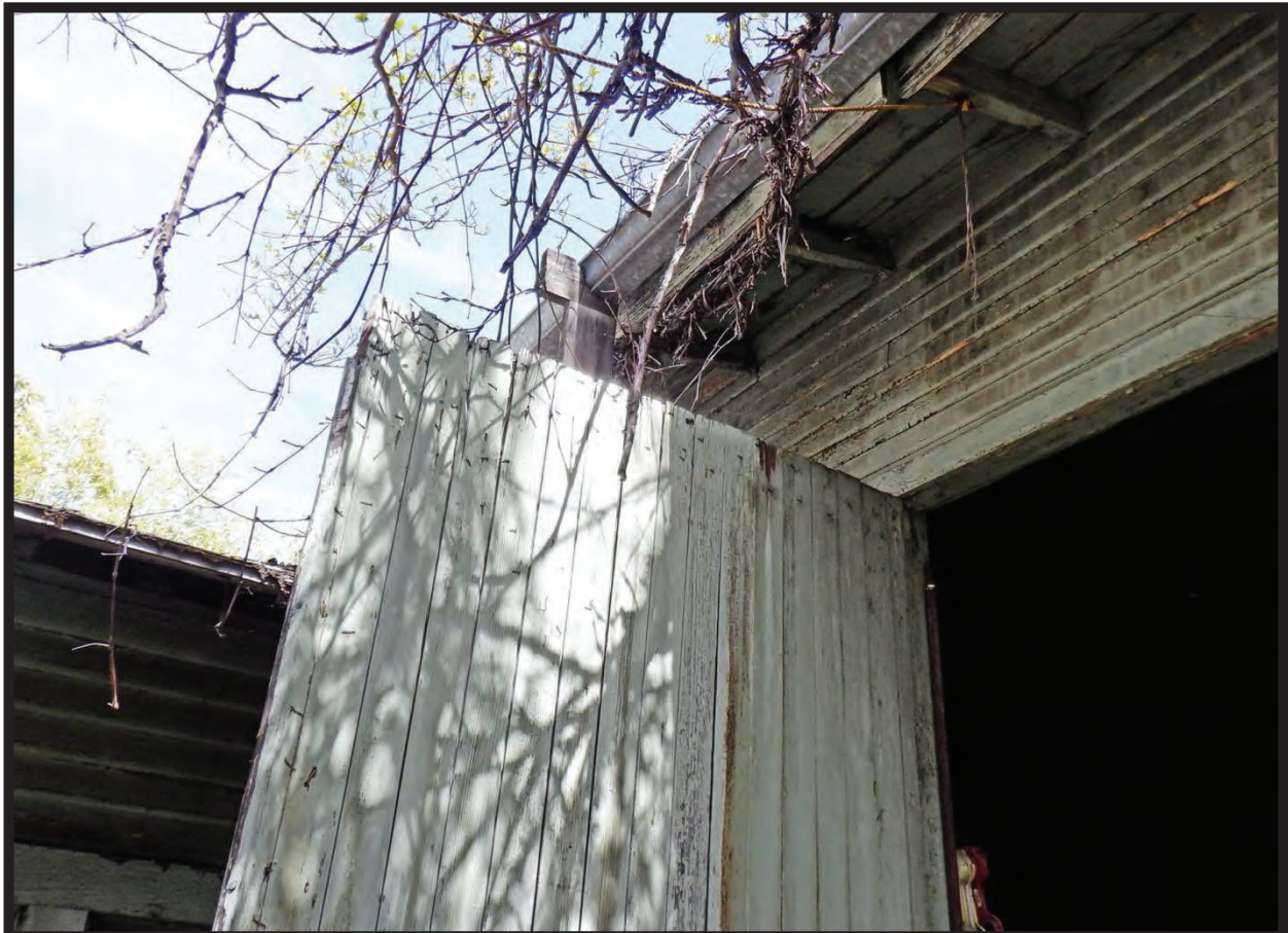
West Elevation of Large Barn/Workshop, 1022 La Cadena Avenue, Arcadia, CA (NNE)
