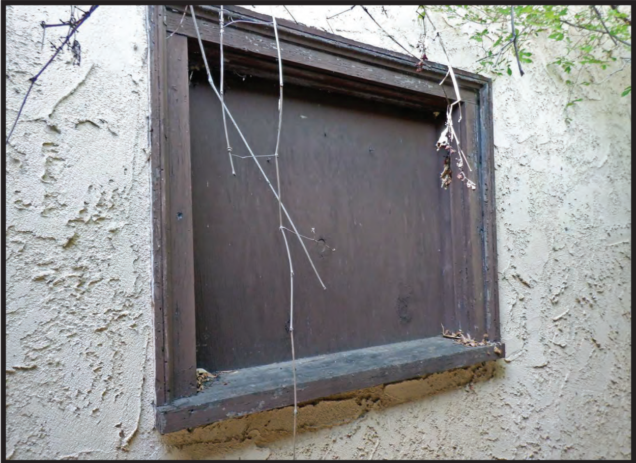
Detail, East Elevation of 1926-1927 Garage, 1022 La Cadena Avenue, Arcadia, CA (NW)
