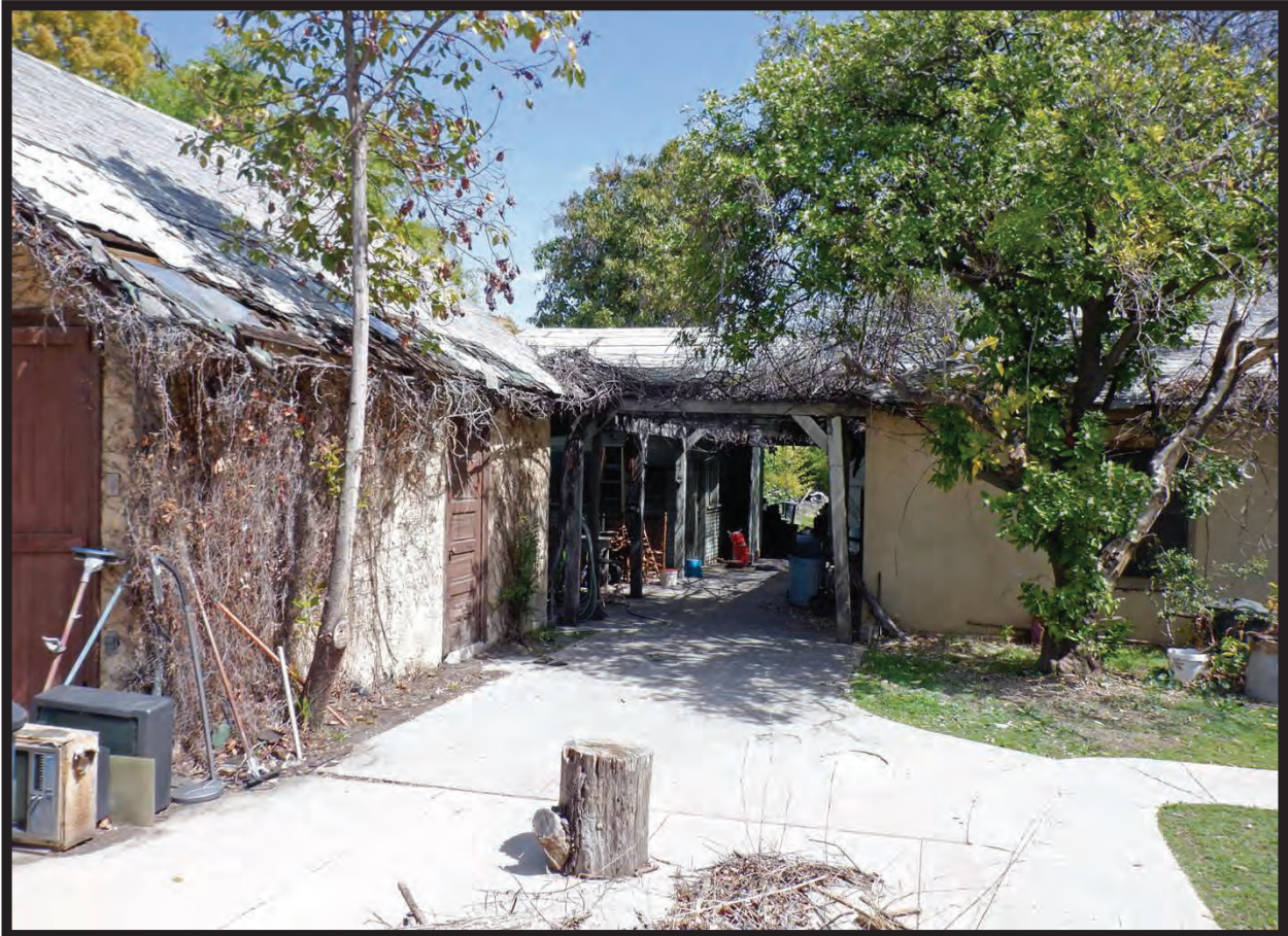
Garage, Second Residence, and Covered Access to Barn/Workshop, 1022 La Cadena Avenue, Arcadia, CA (ENE)
