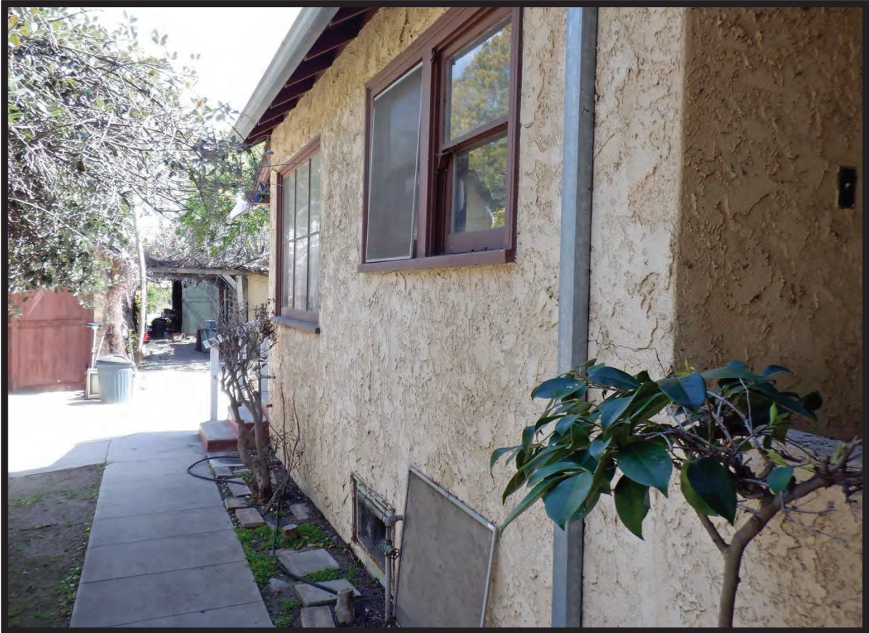
North Elevation of Residence at 1022 La Cadena Avenue, Arcadia, CA (ESE)
